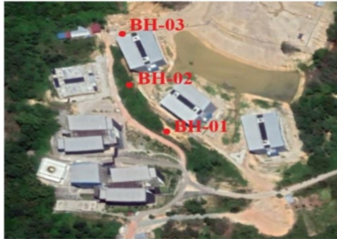
Source : Sampling point for soil analysis (Google Earth, 2020)
