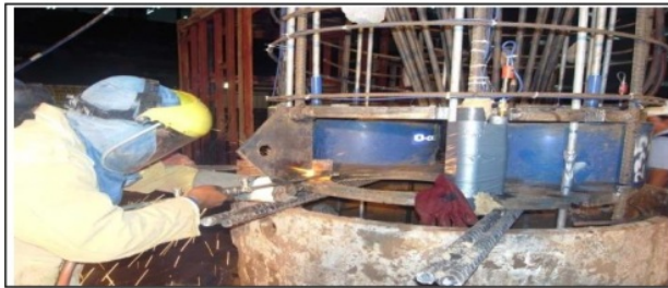
Figure 2. Hydraulic Jack Osterberg Cell.
