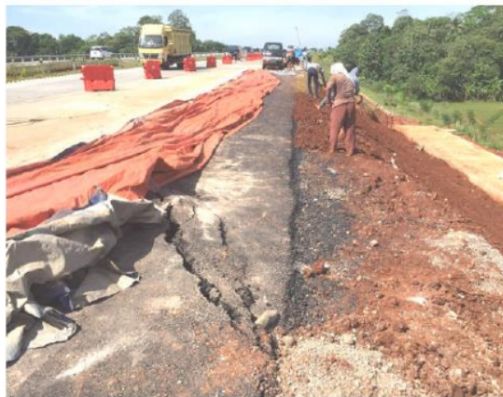
Figure 4. Crack Position
